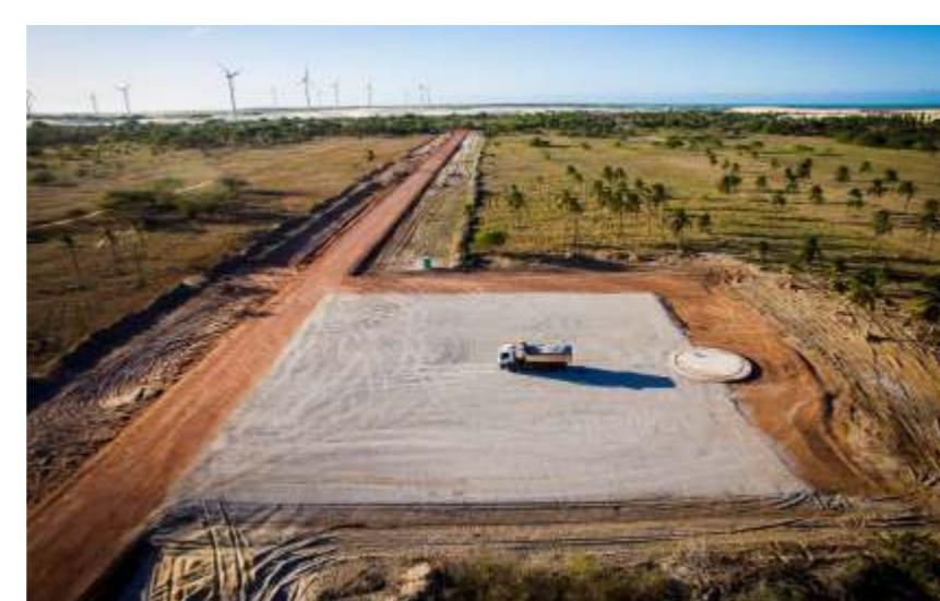
Figure 3. Road access and tower foundation.
